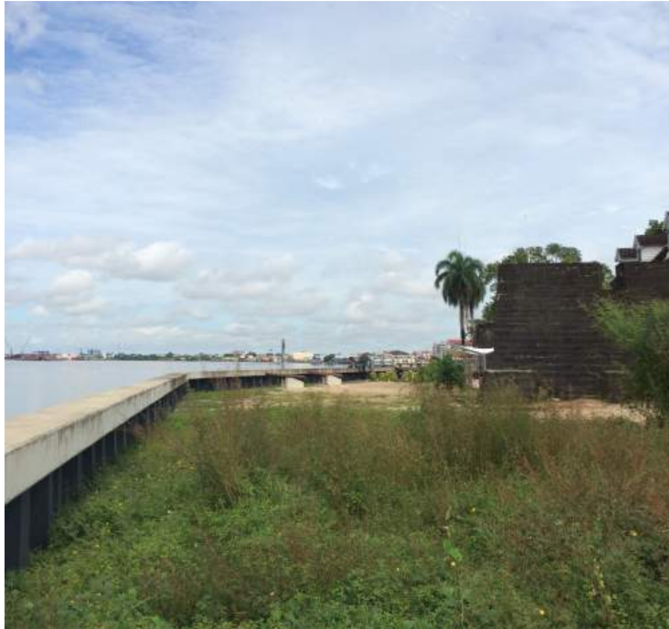
View of the retaining wall at Fort Zeelandia.
